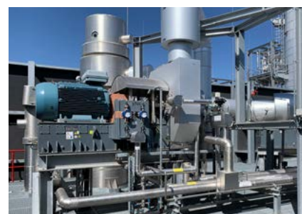
PILLER High-Performance Blower in the bio-ethanol plant
